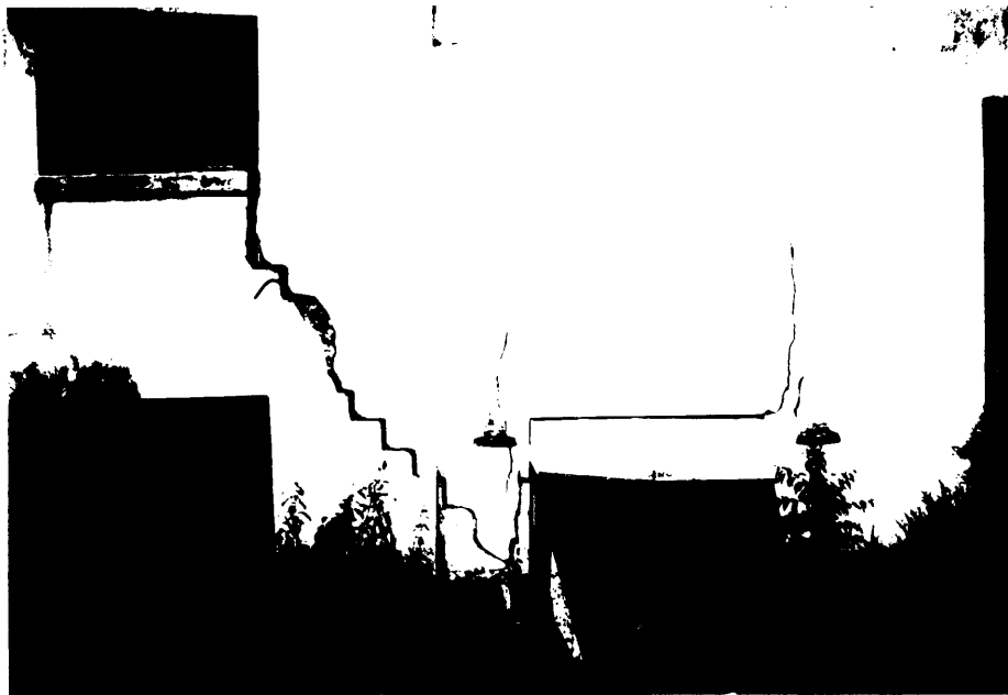
b. Diagonal and vertical cracks
